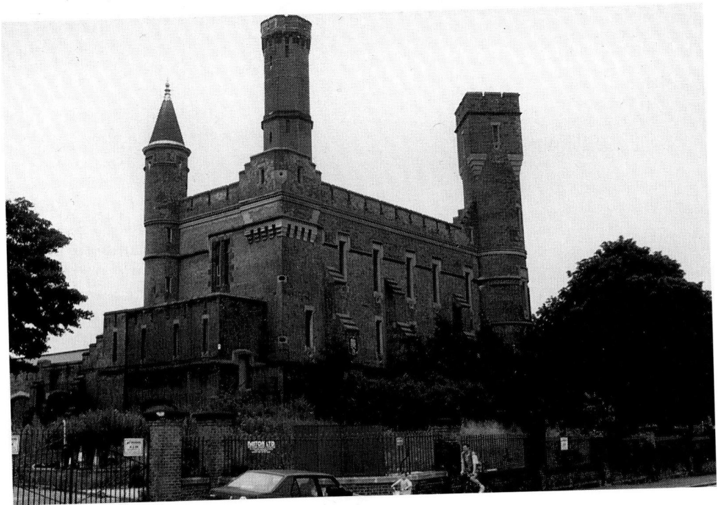
Fig. 10 Green Lanes Pumping Station, Hackney, Grade II*. Built 1854-6 to the design of Chadwell Mylne to resemble a medieval fortress
